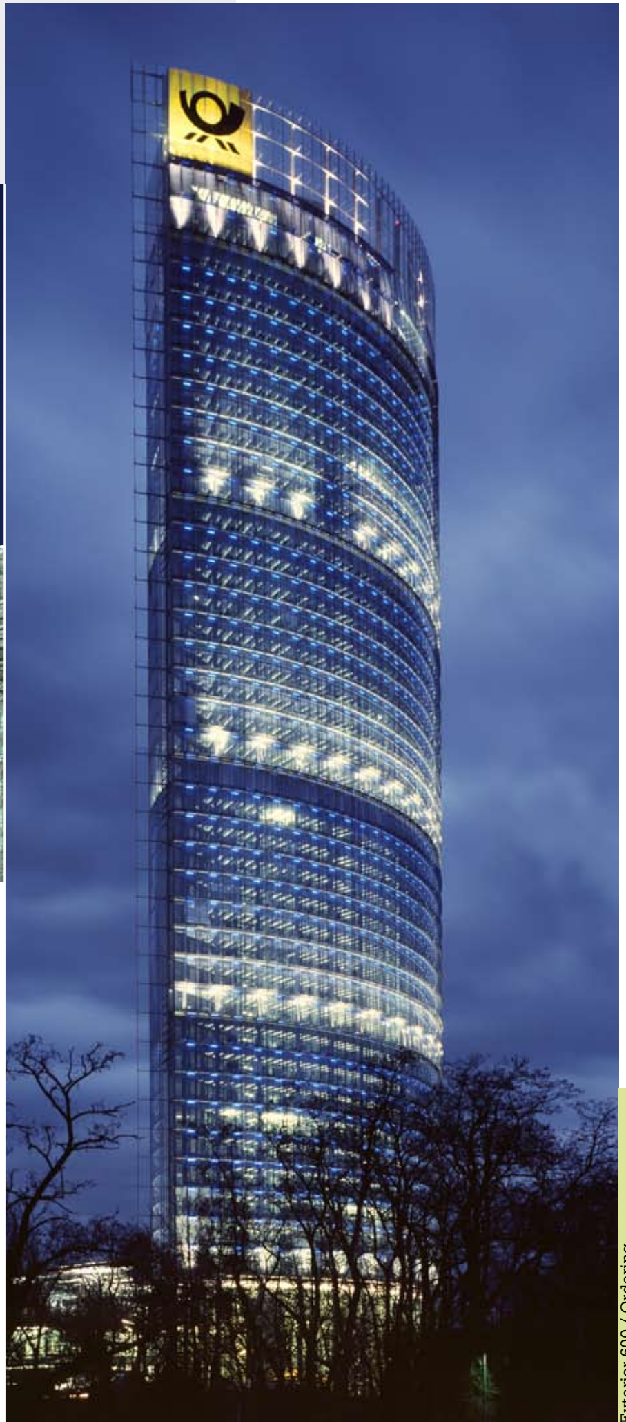
Location: Deutsche Post, Bonn, Germany / Architect: Helmut Jahn, Murphy/Jahn Inc. Designer: Michael Rohde, L-Plan / Light Art: Yann Kersalé
